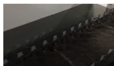
Actiflo® 1 Weir hydraulics maxed out at 120 L/s
