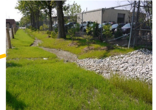
Enhanced Grass Swale
