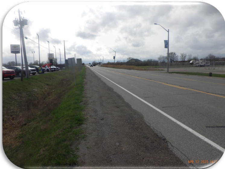
Example of an open municipal drain in Tilbury Fringe – 2023
