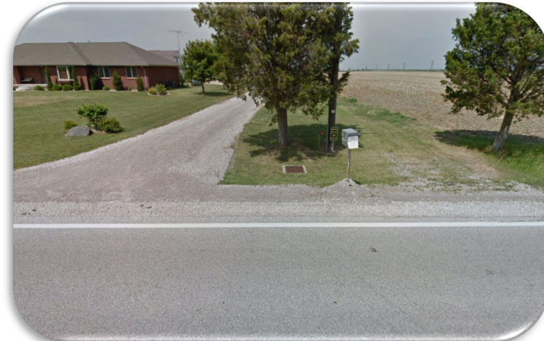
Example of enclosed municipal drain in St. Joachim – 2023
