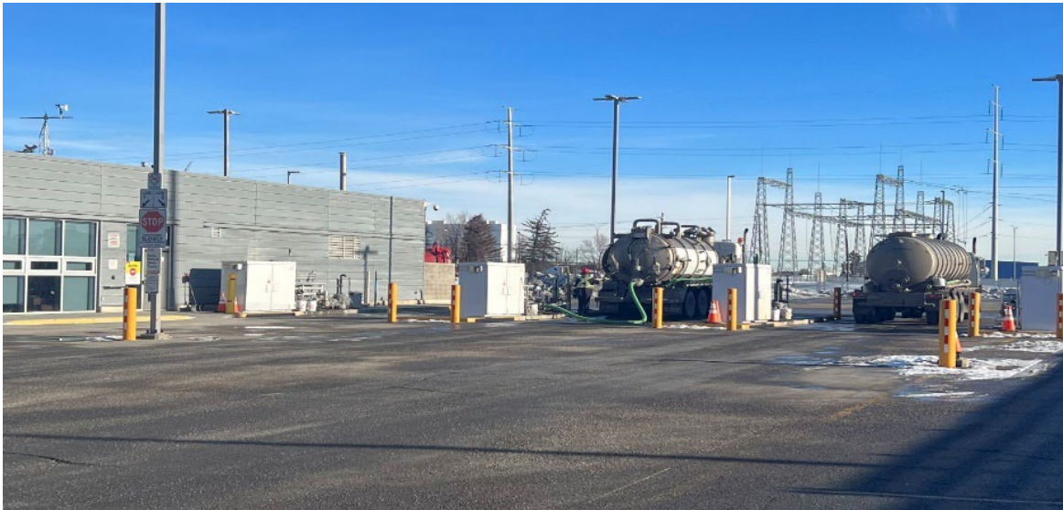
Valleyfield Dump Station
