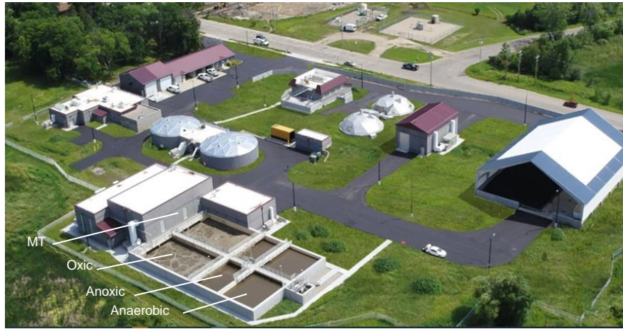
memDENSE installation at Detroit Lakes, MN, USA
