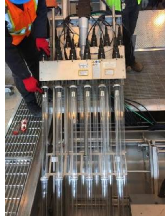
New Lamp Bank: 1,008 Duron Lamps (600W ea.)
