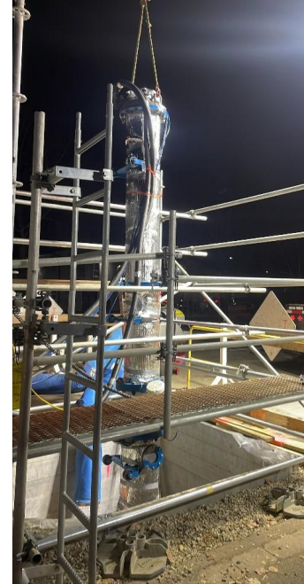
Wet tap with launch tube (left) and insulated retrieval/extraction tube (right)
