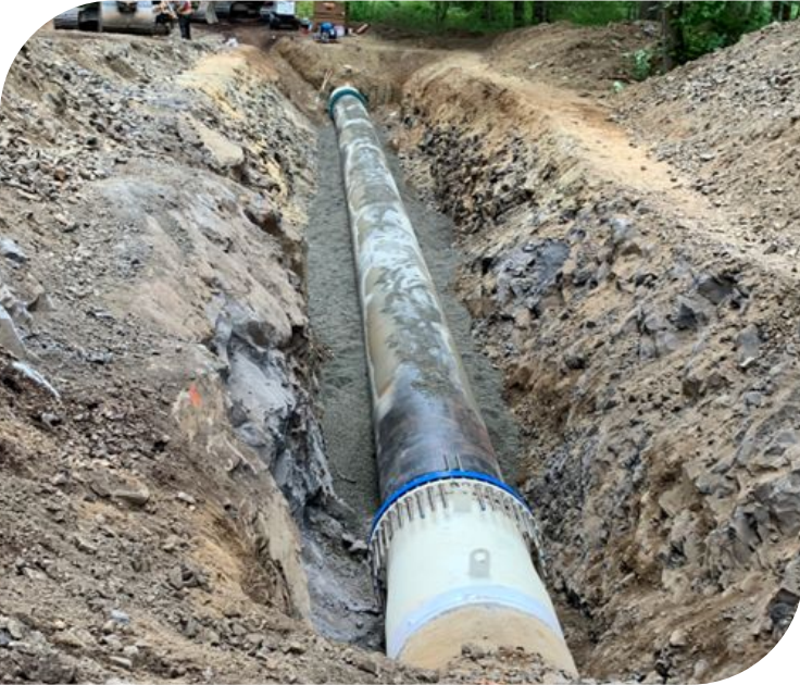
In-line Pipe Replacement
