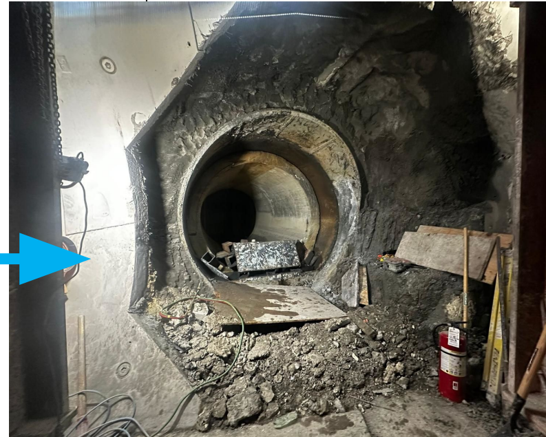
Removal of PCTL & Locating Previously Installed Adit
