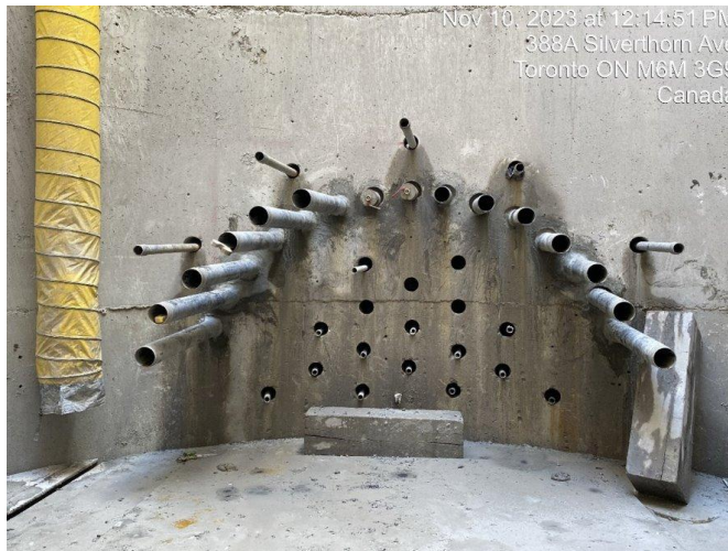
Ground Consolidation (From Drop Shaft)
