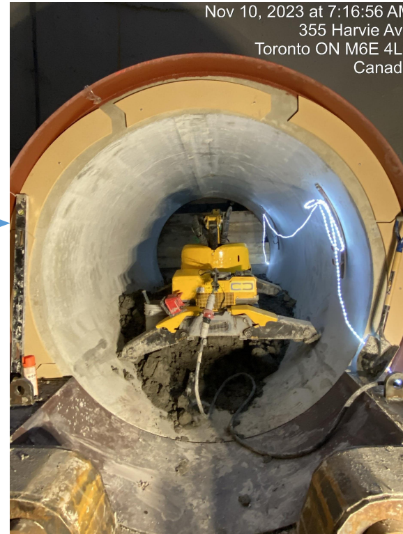
Hand Mining (Pipe jacking from Drop shaft to few metres away from proposed tunnel alignment)
