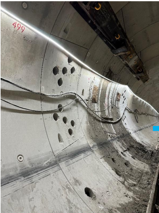
Ground Consolidation w/ Grout Injection
