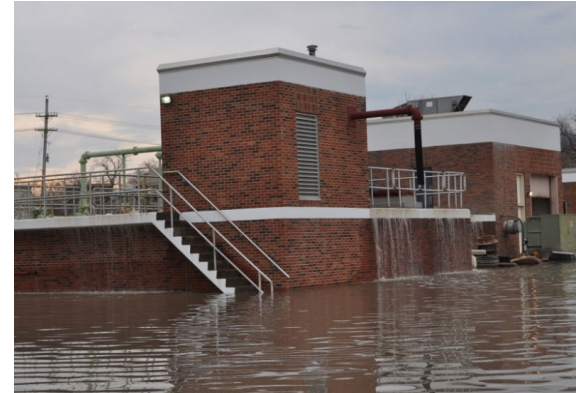
Overflow at the Plant
