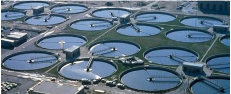
"Sewage treatment plant" by Chesapeake Bay Program is licensed under CC Attribution 2.0 Generic (CC BY 2.0)
